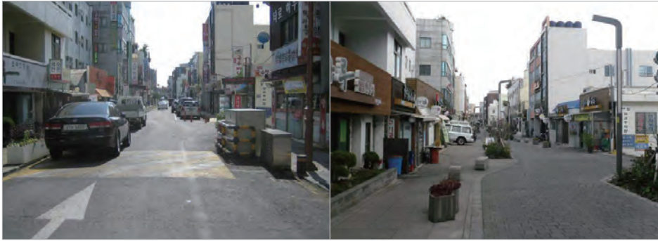
Figure 2.2 Before and after pedestrian priority zone construction
